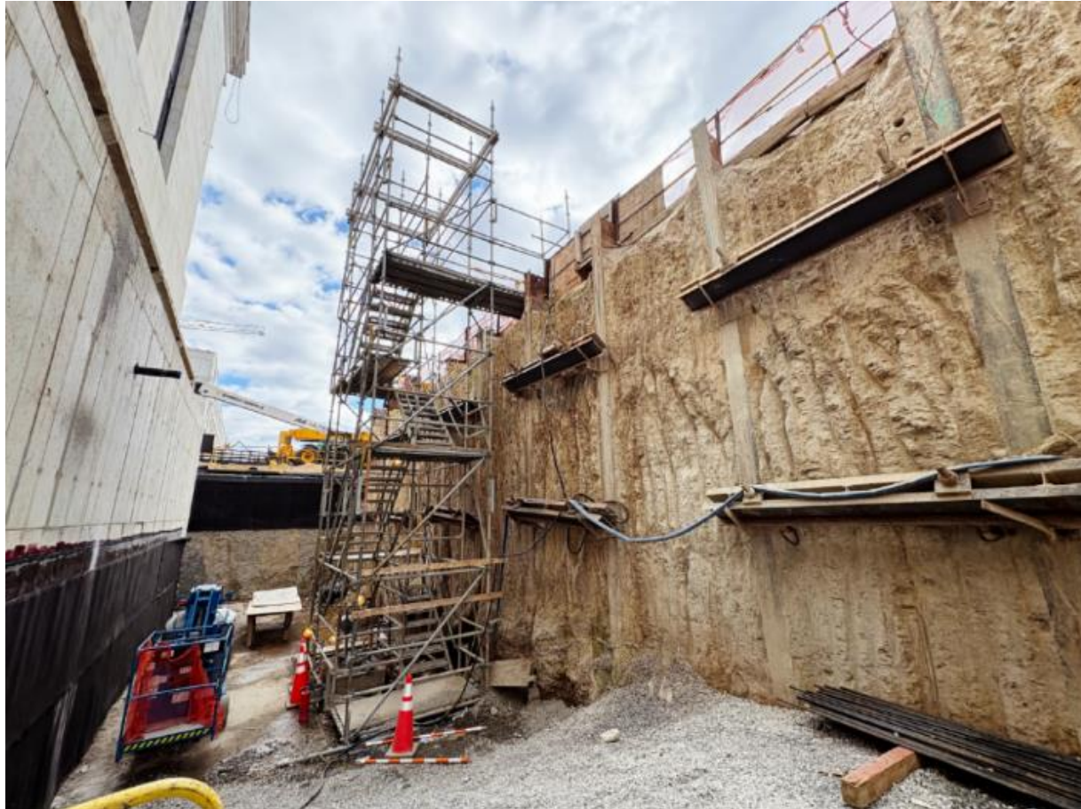
Figure 6. Excavation Work for the Eccles Building
