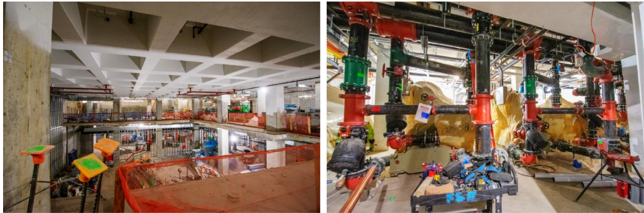
Figure 8. New Underground Conference Area (Left) and New Utility Plant Beneath 1951 (Right)
